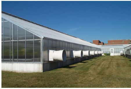
Fig. 1 Axial ventilation fans in greenhouse applications
